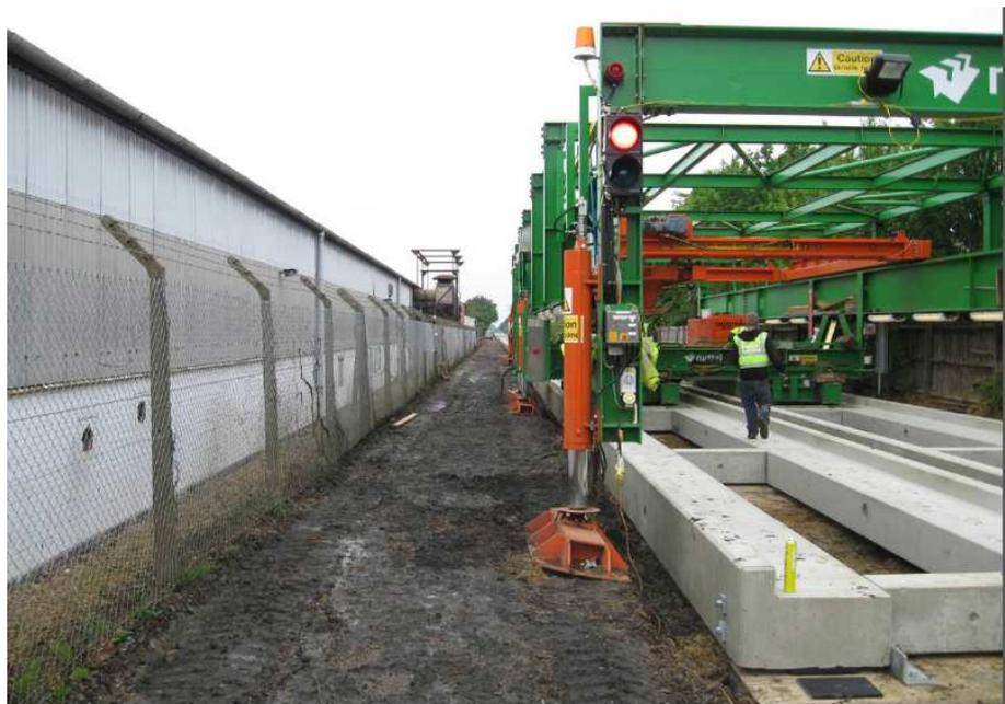
**Figure 2 – Gantry Laying PCC Units**
